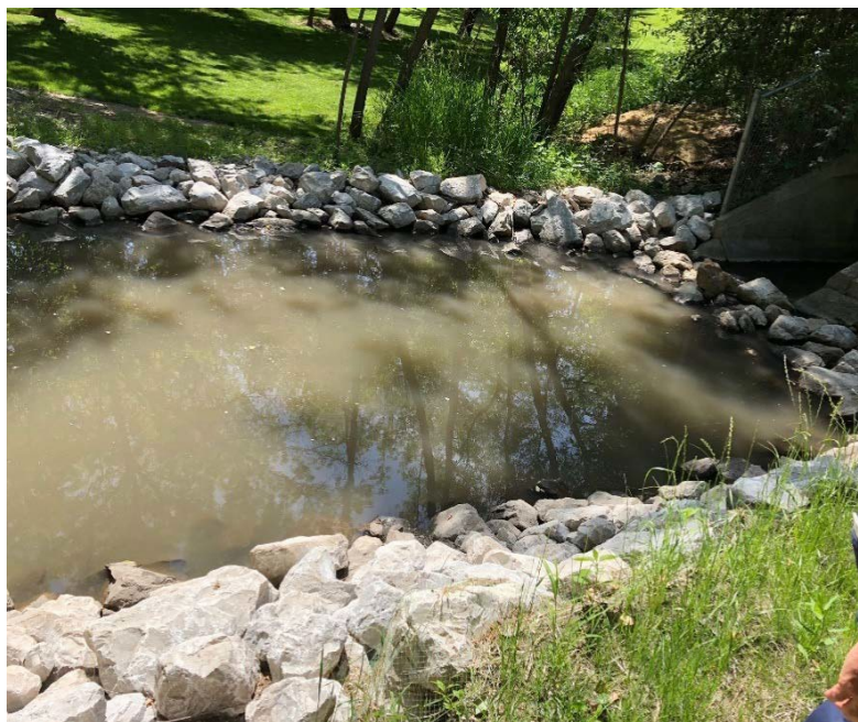
Example of a Riprap Stilling Basin
