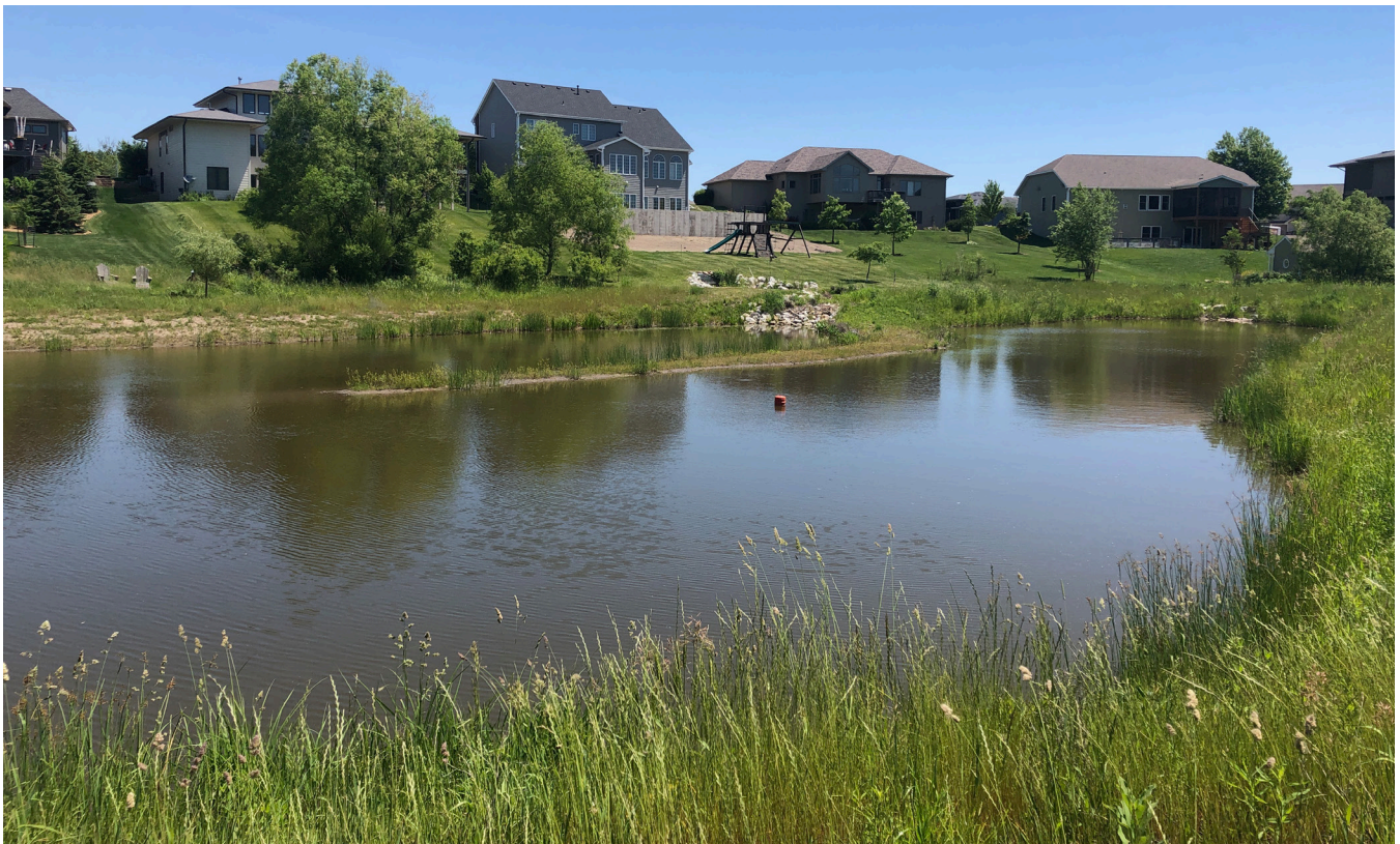
Example of a Stormwater Detention Basin Retrofit in Clive, IA. Photo Source: Walnut Creek WMA.
