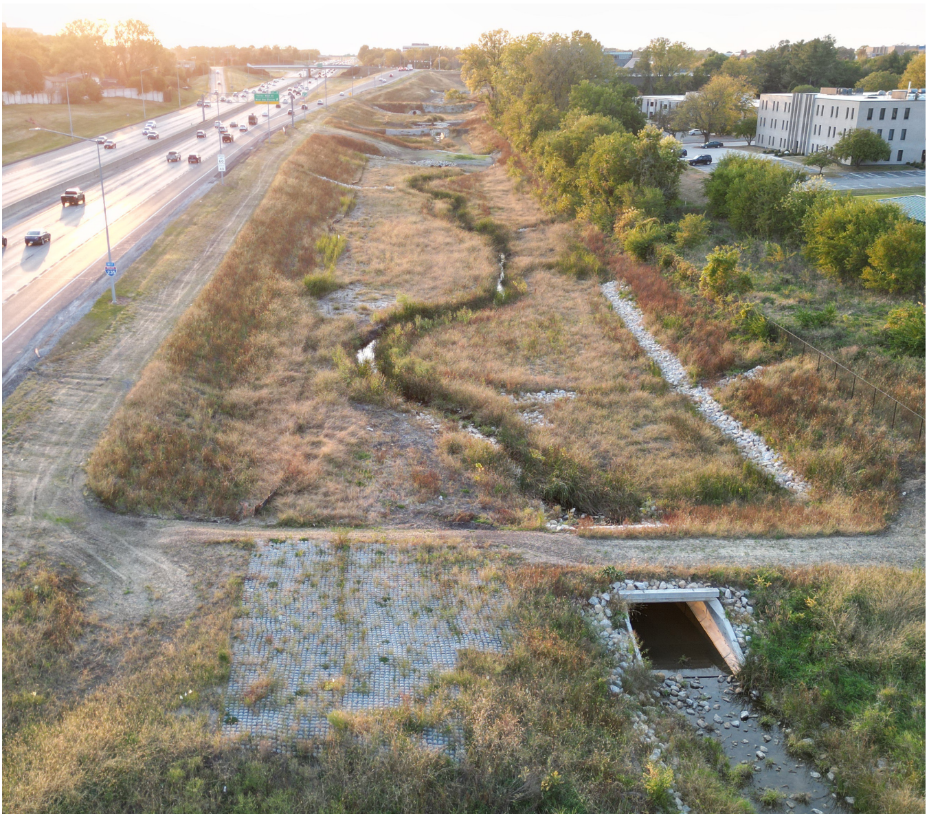
Blue Creek Stabilization in West Des Moines. Source: Author.
