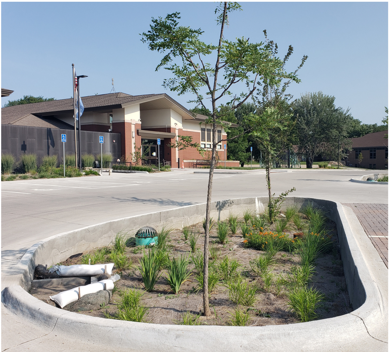
Waukeee Library Bioretention Cell. Source: Walnut Creek WMA.
