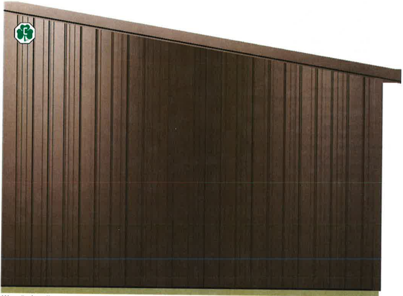
West End Wall 1 on Building 1
