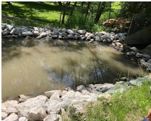
Example of a Riprap Stilling Basin
