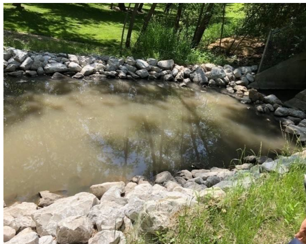
Example of a Riprap Stilling Basin
