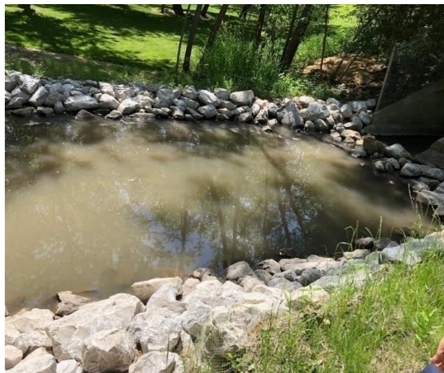
Example of a Riprap Stilling Basin
