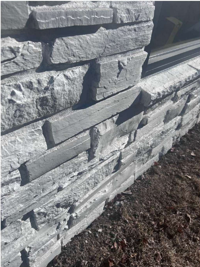
Close-up of treatment application on building stone
