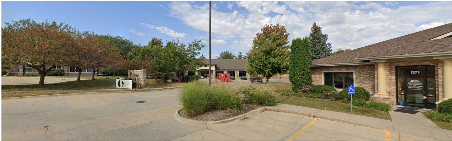
Subject property and adjacent commercial properties prior to exterior updates
