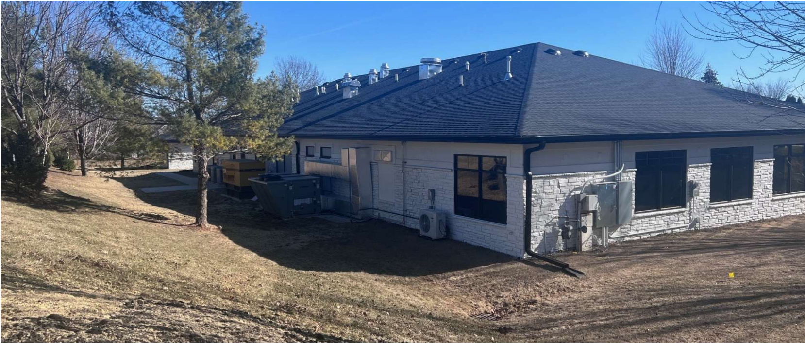
Back of building from top of berm facing southeast
