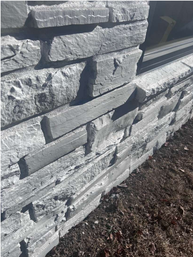
Close-up of treatment application on building stone
