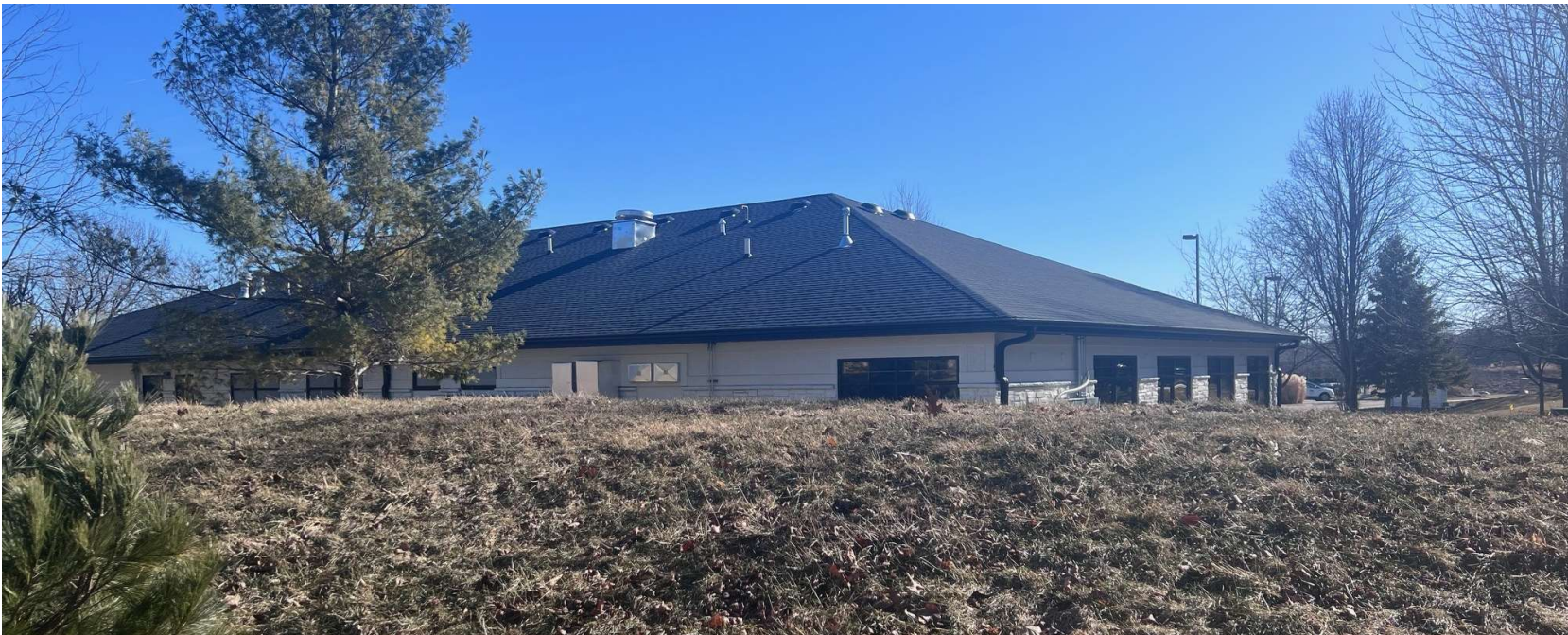
Back of building from residential properties to the north
