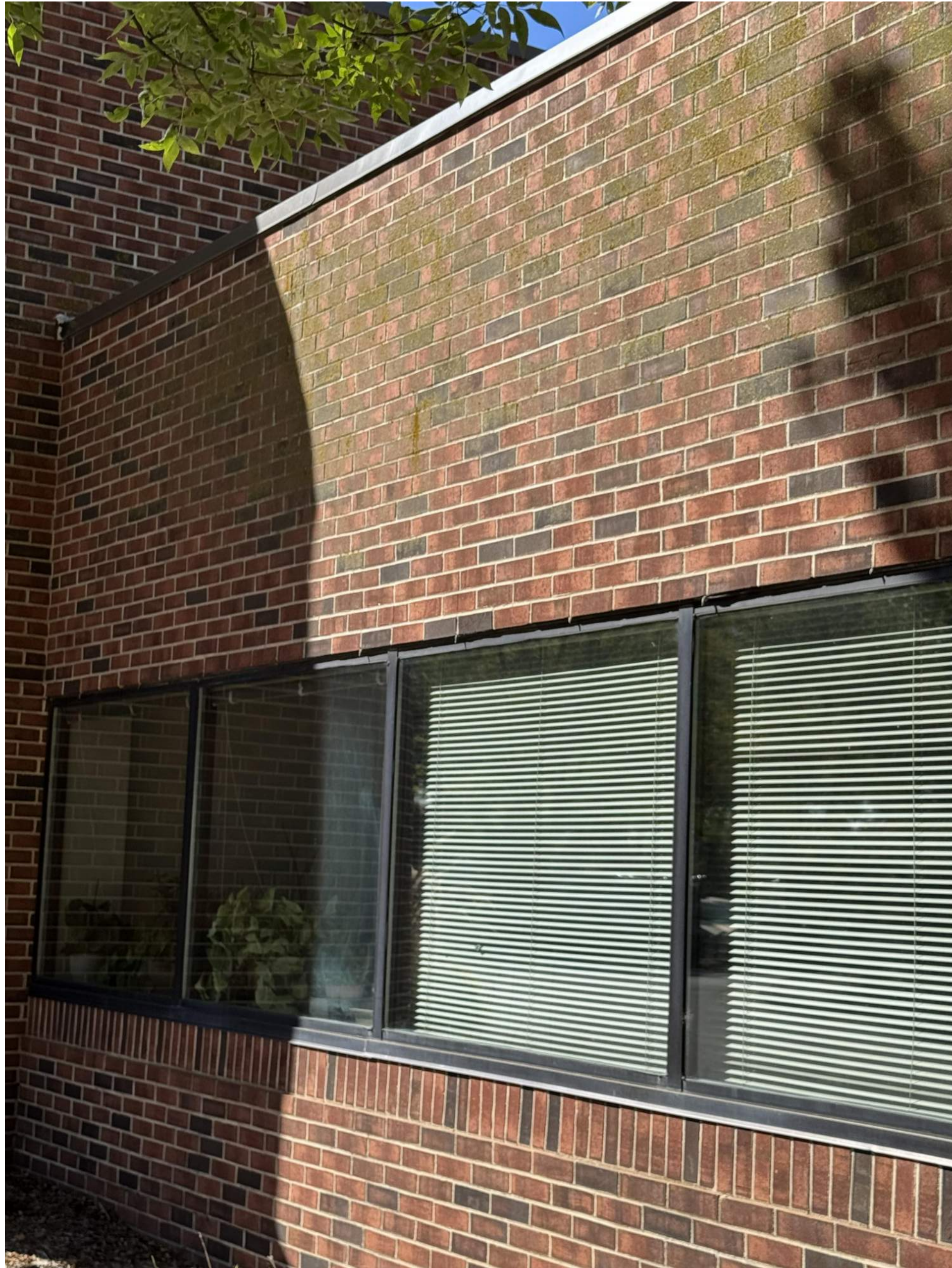
EXAMPLE OF ORGANIC GROWTH ON BRICK NEAR PARAPET
