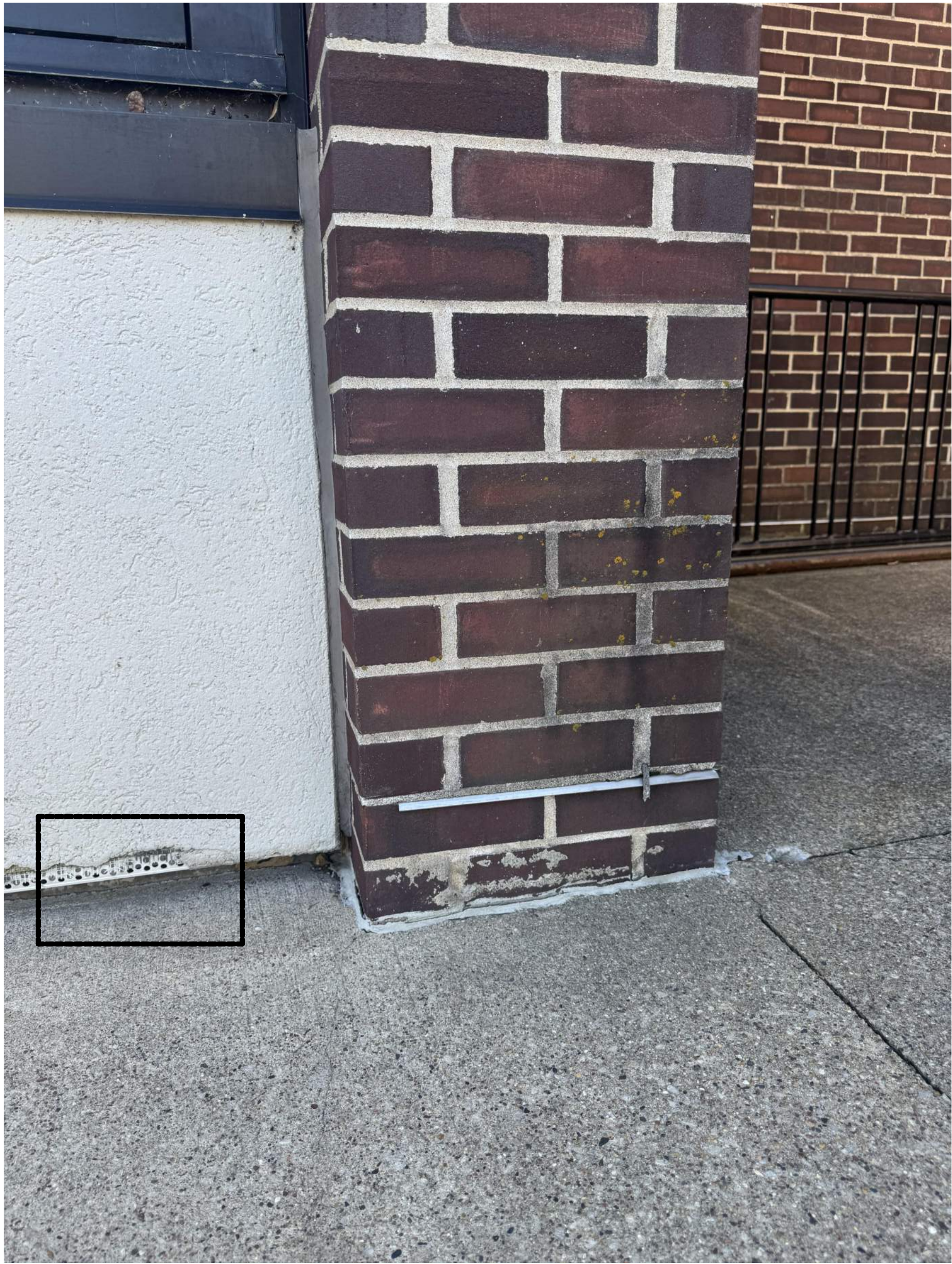
AREA OF EIFS DETERIORATION AT LIBRARY ENTRY
