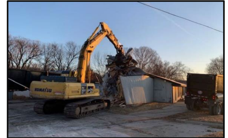
2019 HMGP Acquisition and Demolition
